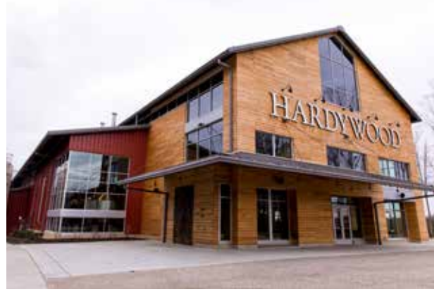
Hardywood West Creek 820 Sanctuary Trail Drive Neighborhood: Henrico Owner | Developer: Eric McKay and Patrick Murtaugh Architect: Price Simpson Harvey Contractor: Loughridge & Co. Landscape Architect: Waterstreet Studio Interior Designer: Graphite + Co.
