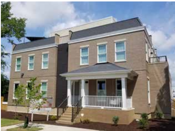
Jefferson Green Condominiums 1902 - 1904 - 1906 Princess Anne Avenue Neighborhood: Union Hill Owner | Developer: Richard Cross, Hollyport Ventures LLC Architect: R. Michael Cross Design Group Contractor: Health-E Community Enterprise of Virginia Inc.
