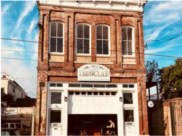
Ironclad Coffee Roasters Café 1805 East Grace Street Neighborhood: Shockoe Bottom Owner | Developer: Bruce Vanderbilt Engineer: John Spence Contractor: CB Chandler Construction Designer: Caroline McIlraith/ Chyrelle Dorinsky
