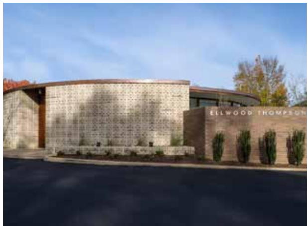
The Round Building 3540 Floyd Avenue Neighborhood: Museum District Owner: Rick Hood Architect: Walter Parks Architects Engineer: Dunlap and Partners Contractor: J.A. Heisler Construction Landscape Architect: Four Winds Design Tax Credit Consultant: Sadler & Whitehead Architects
